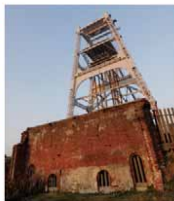
Steel shaft tower
